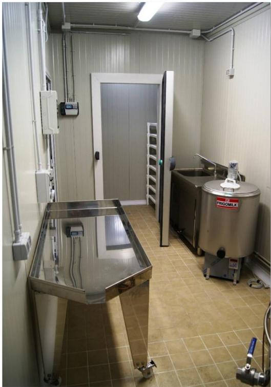
*The mobile dairy is made up of: refrigerated tank for milk storage, multifunction for pasteurization and heating of milk, stainless steel processing benches, refrigeration chamber for cheese storage.*
